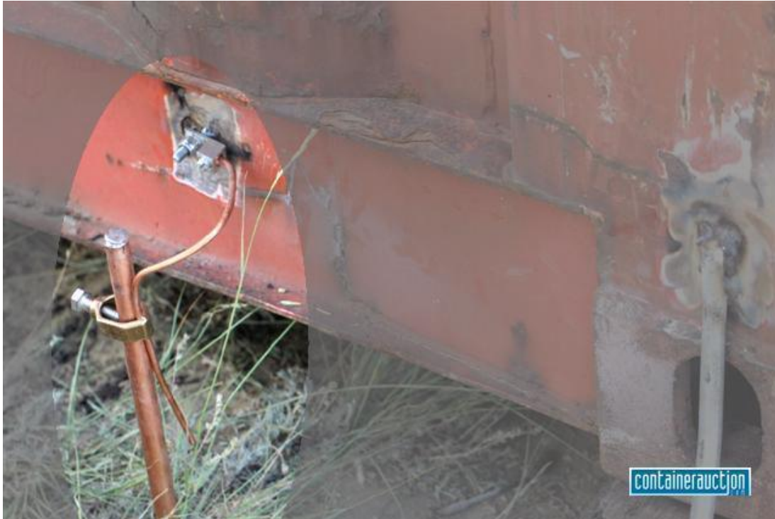
FIGURE 2 EARTHING ROD CONNECTED TO CONTAINER
