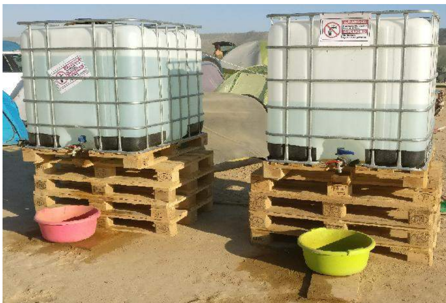
FIGURE 3: WATER CUBE STAND USING PALLETS
