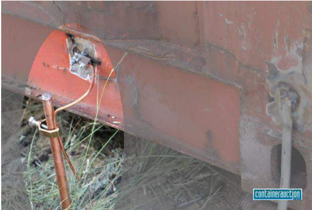
FIGURE 4: EARTHING ROD CONNECTED TO CONTAINER
